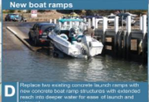
**D** Replace two existing concrete launch ramps with new concrete boat ramp structures with extended reaches into deeper water for ease of launch and retrieval.
