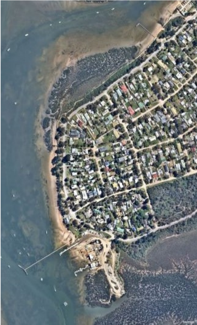
Aerial photo of the Warneet Boating Precinct area
