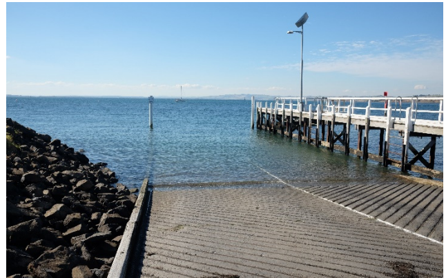
Figure 5: Boat Ramp in Newhaven, Victoria
