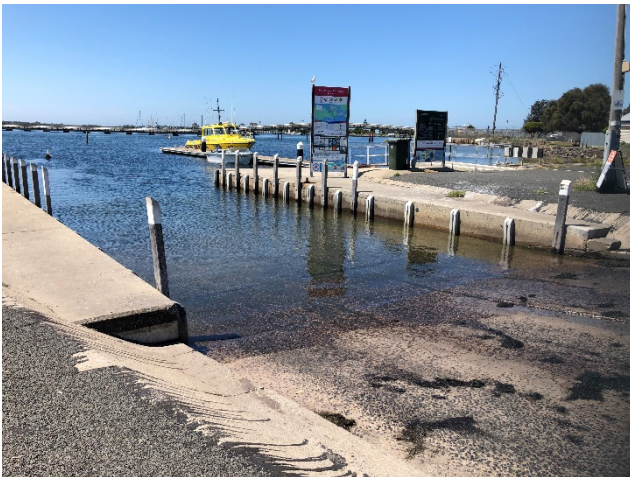
Figure 4: Boat Ramp in Queenscliff, Victoria
