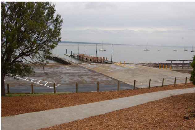
Figure 3: Boat Ramp in Corinella, Victoria
